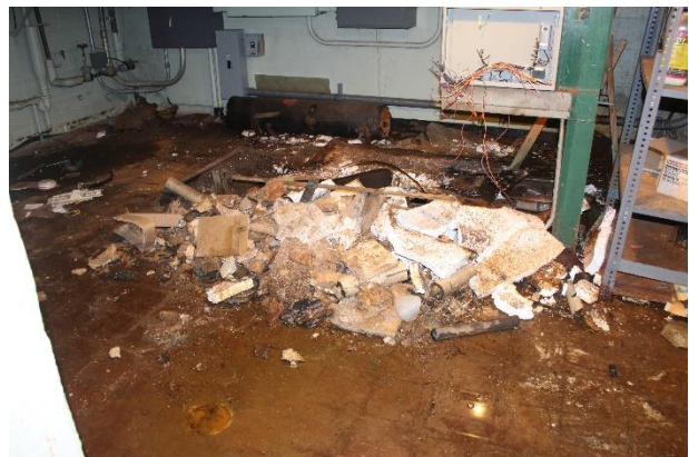
Figure 21: Continuing water infiltration and associated damage is a major concern.
