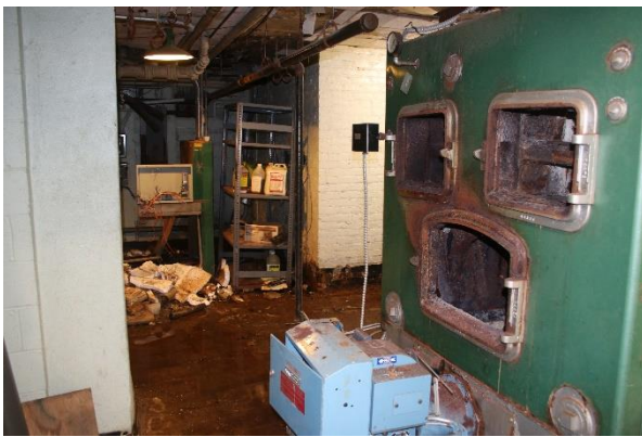
Figure 20: The cast iron doors have been removed from the old furnace.
